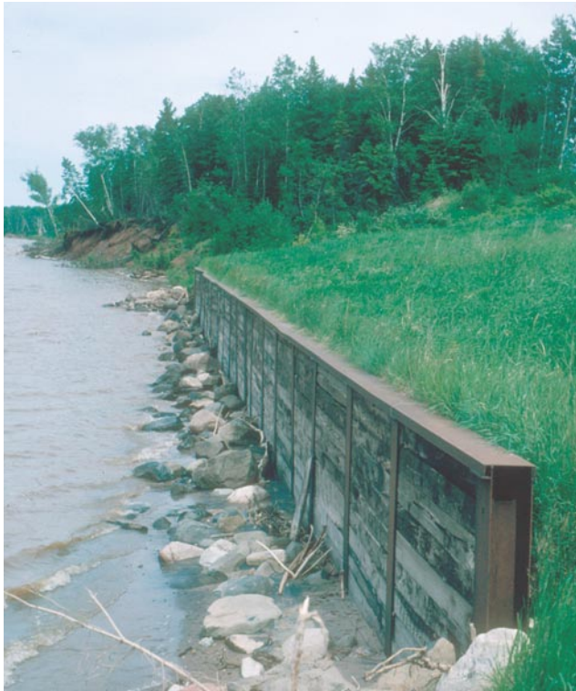
Seawall on Lake Superior
